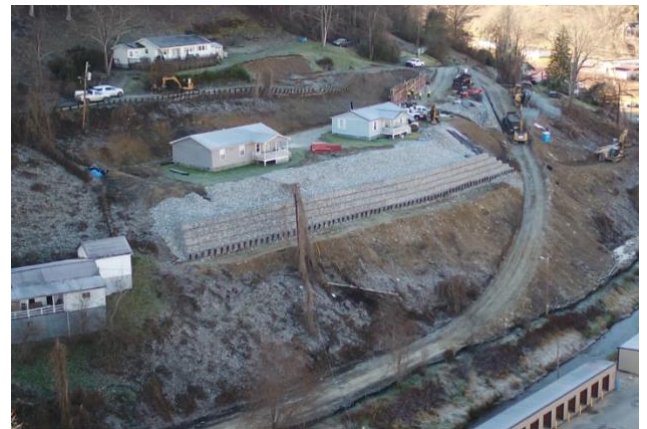
Reclamation of severe landslide in Eastern Kentucky
